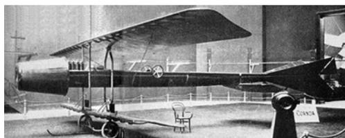
Fig. 1 In 1910, Henri Coandă built and flew the world's first jet aircraft
