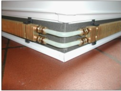
Fig.9 Water plinths mounting in a house corner
