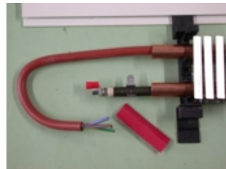
Fig. 7 Electrical plinth mounting in a house
