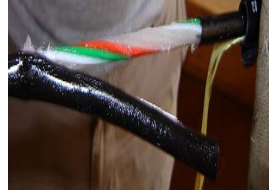
Fig. 3 – Eliminating the inner liner of fiber cable protection
